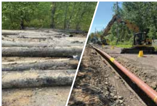
Oilwell Road: Old pipe replaced with new.
