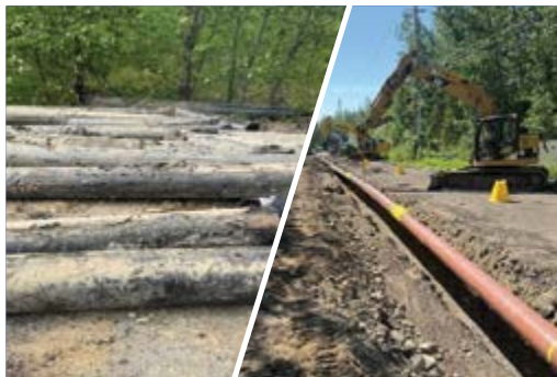
Oilwell Road: Old pipe replaced with new.
