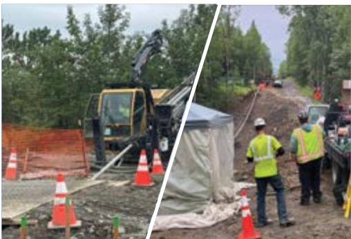
Westside Feeder: Horizontal drilling took place beneath the New Seward Hwy. and Rabbit Creek. This project will retire ~14,000 ft. of 50-yr-old pipe.
