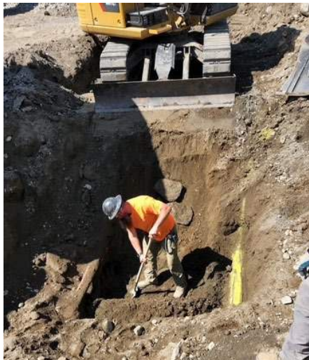
Photo Credit: Brent Billingslea of GMC Contracting, Inc.
