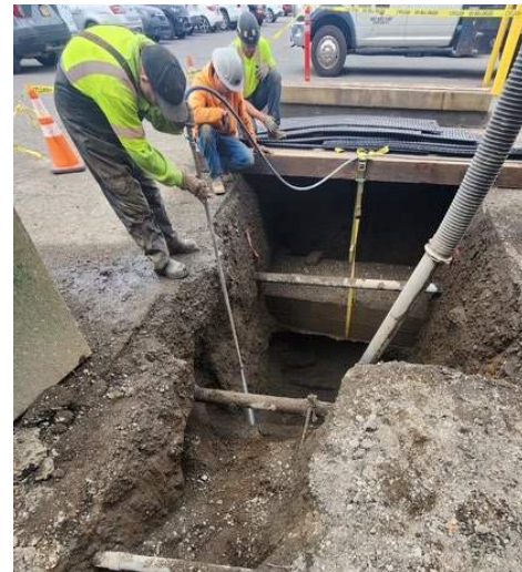
Photo Credit: Precision General Contractors
